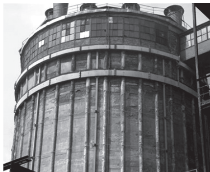
Fig. 6. a) damage of prefabricated shell elements four years after repair; b) exhaust chimney near the tower
