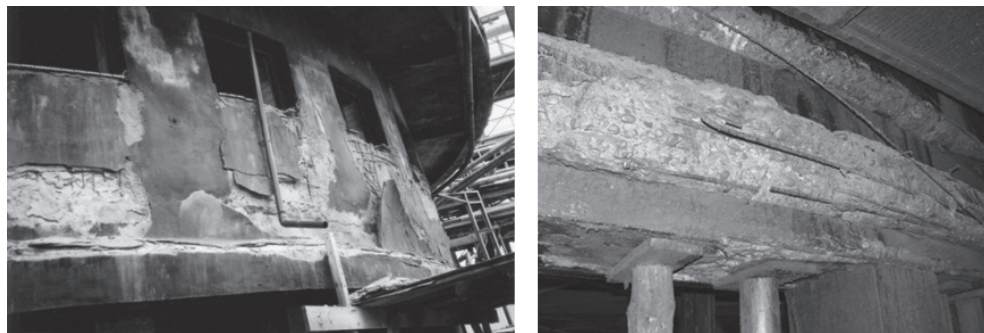
Fig. 3. Corrosion of monolithic foundation of the tower in 2002
