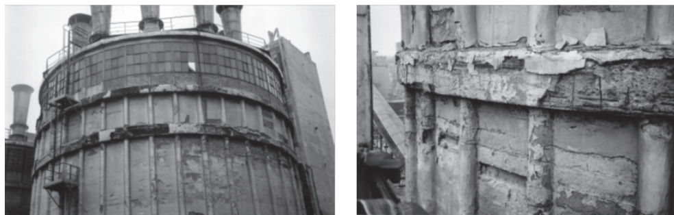
Fig. 4. Corrosion of the prefabricated cylindrical shell (2002)
